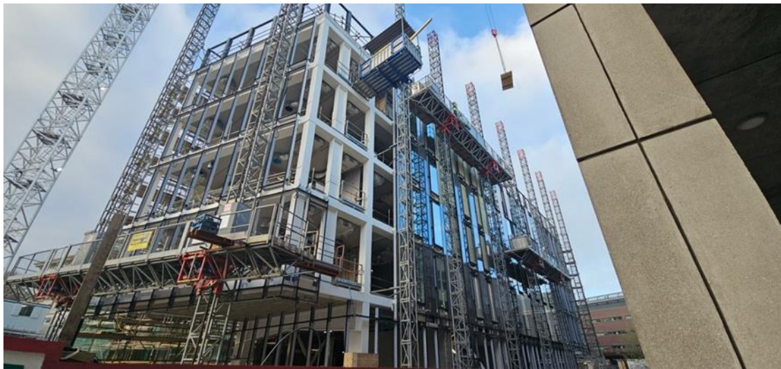
Figure 1. 2 Building Façade work in progress at TCD 2024
