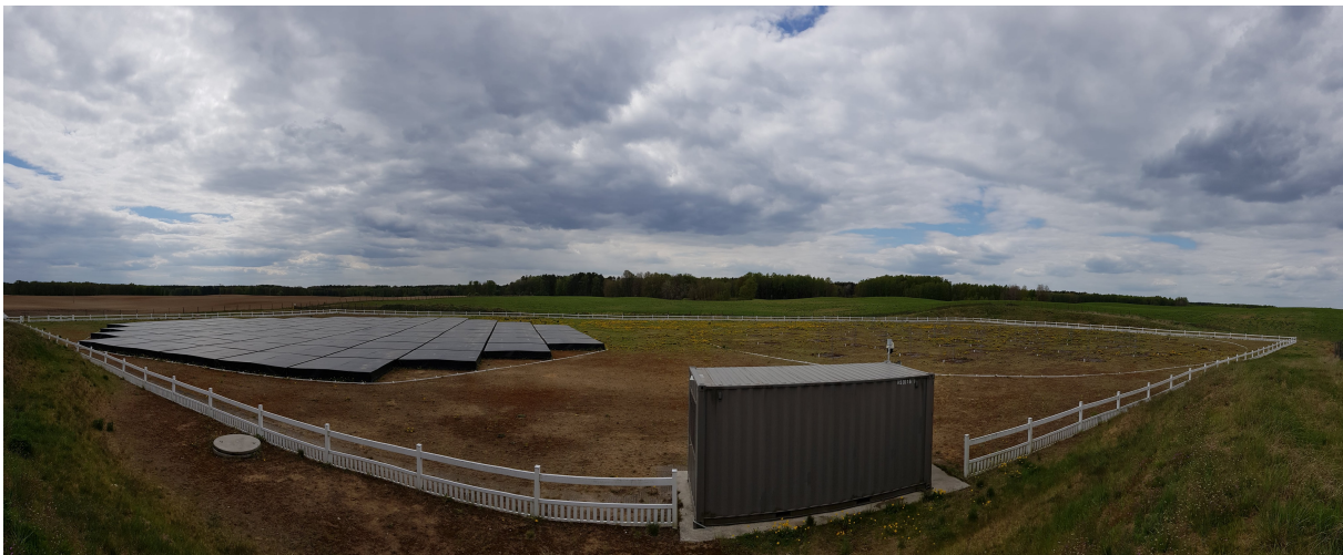
Figure 1: The LOFAR station in Baldy near Olsztyn. HBA (High Band Antennas) part is placed on the left, and LBA (Low Band Antennas) part can be seen on the right. A container with back-end instrumentation is shown in the middle
