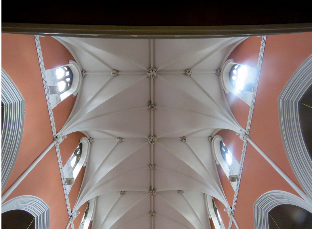
Plate 5: The nave vault of St Patrick's Pro-Cathedral, Dundalk.
