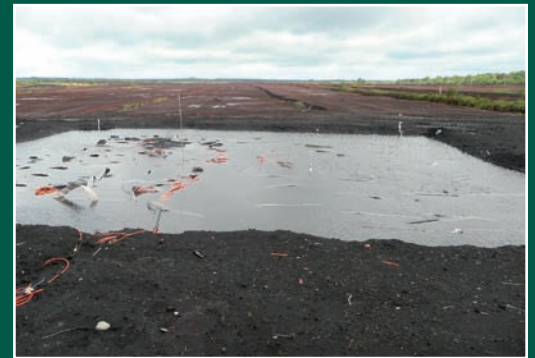
A before and after shot showing the effects of vacuum consolidation to accelerate the flow of water from the peat
