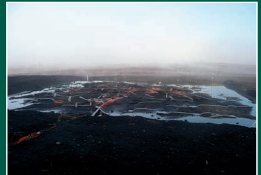
A before and after shot showing the effects of vacuum consolidation to accelerate the flow of water from the peat
