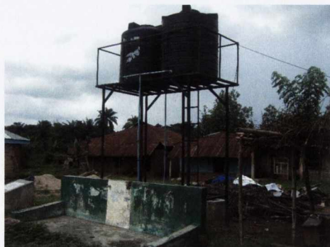
Plate 4.6 Boreholes within the community (Photo: Síle Molloy)
