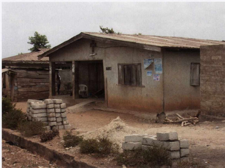
Plate 2.4 Typical village house with concrete walls and corrugated iron roof (Photo by: Síle Molloy)
