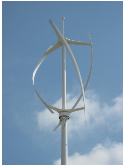
(a) Lift type vertical axis wind turbine on Liverpool waterfront [14].
