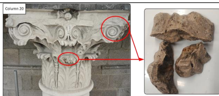
Figure 2. Portland stone at The Four Courts showing old mortar repairs made with crushed Portland stone - figure 3.
