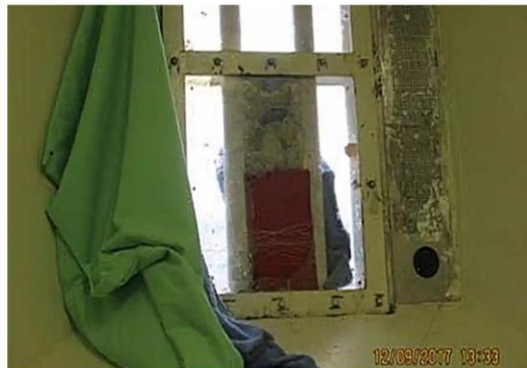
▲ A broken window in a cell at HMP Liverpool in September 2017 when inspectors conducted a surprise inspection. Photograph: HM Inspectorate of Prisons/PA
