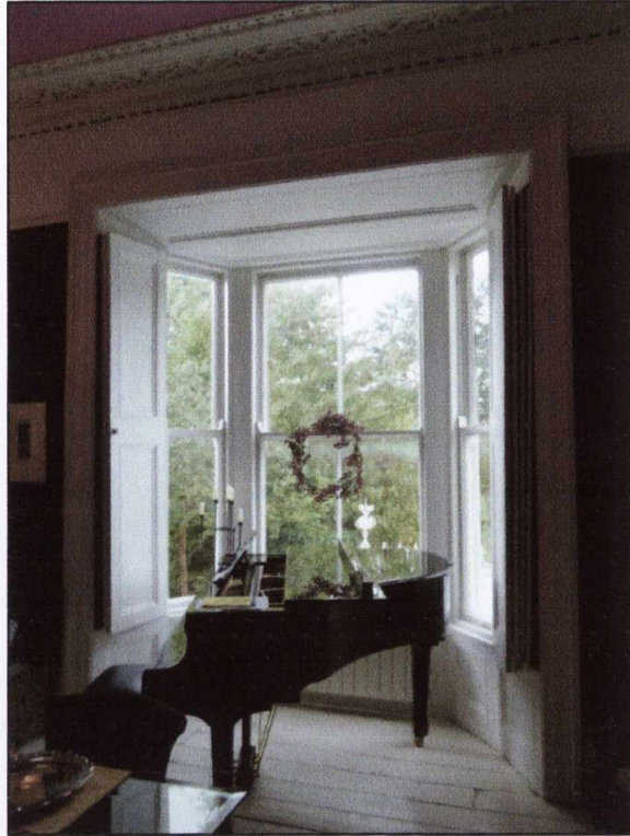
3.117: Number 3 Rostrevor Terrace: bay window to rear reception room
