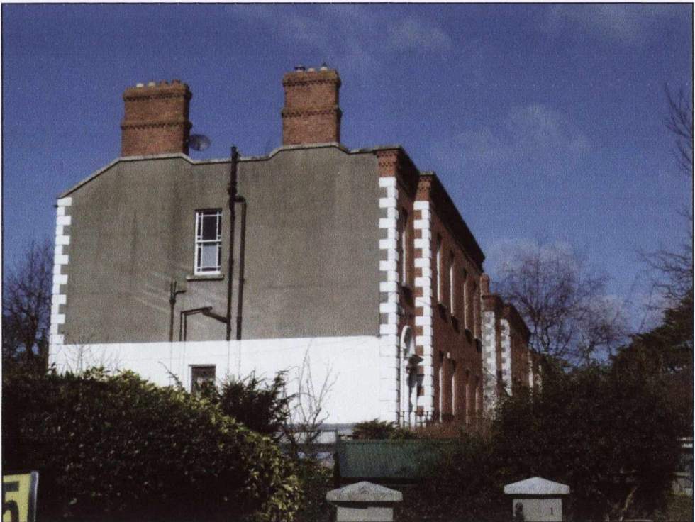
4.10: Number 14 Rostrevor Terrace: detail of end wall.
