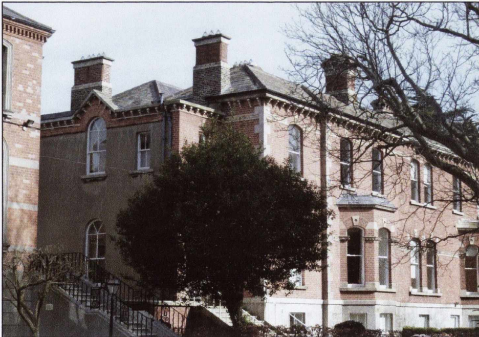
3.105: Number 4 Ailesbury Road: detail of side return.
