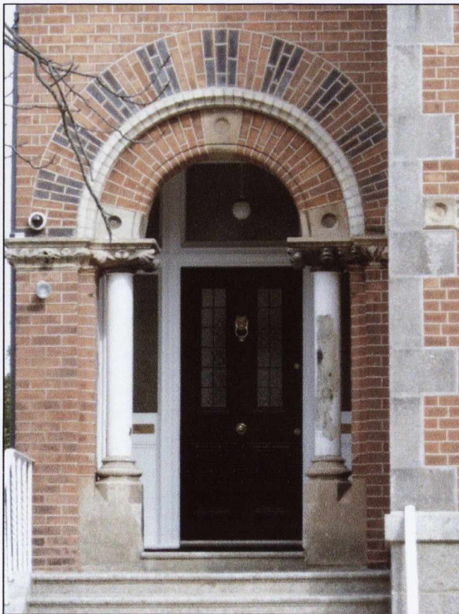
3.110: Number 4 Ailesbury Road: detail of front entrance.
