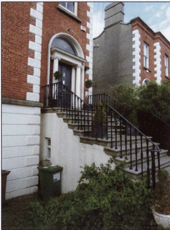
4.28: Number 3 Rostrevor Terrace: detail of entrance steps.
