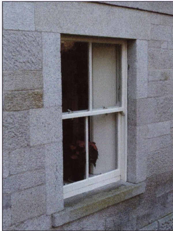
4.32: Number 17 Ailesbury Road: detail of granite facing to the lower level.
