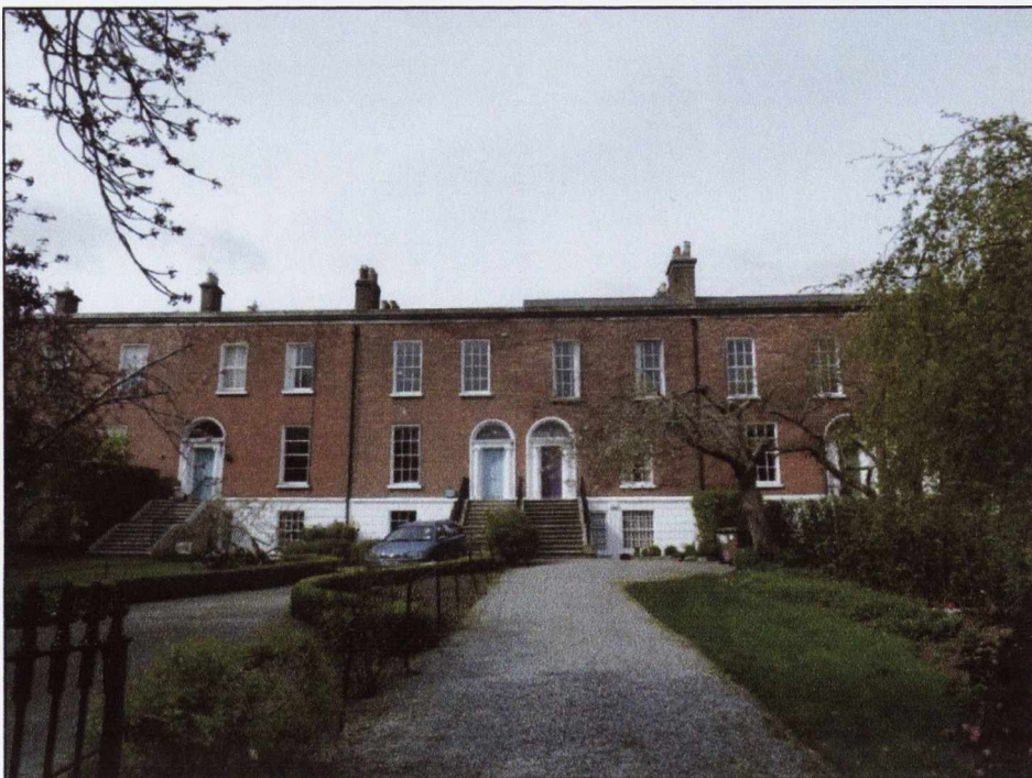
3.80: Wellington Road: west side.
