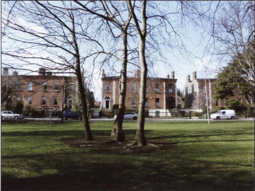
3.111: Rostrevor Terrace, viewed from the Orwell Road.
