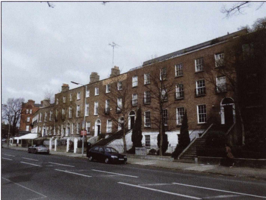
3.2: North side of Pembroke Road
