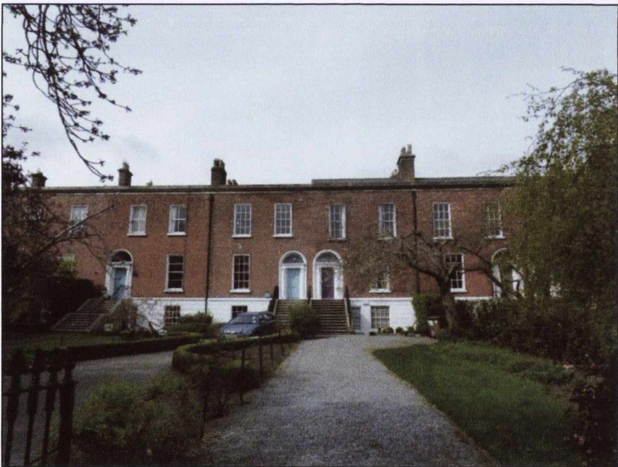
3.5: West side of Wellington Road.
