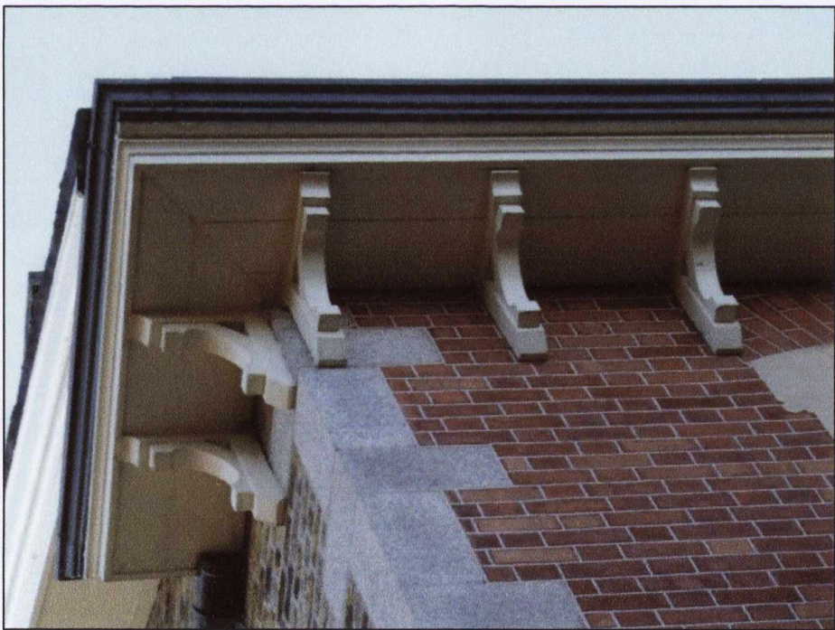
3.101: Eaves brackets to Number 17 Ailesbury Road.
