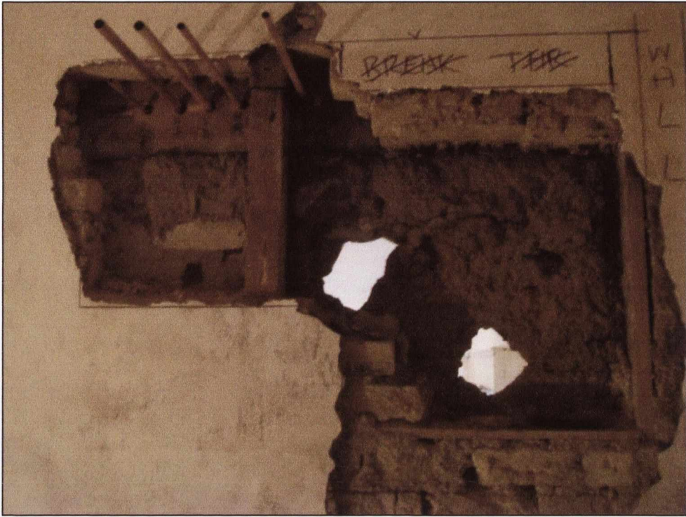
4.23: Number 7 Ailesbury Road: bricknogging partition
