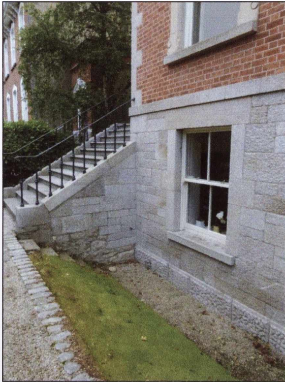
4.27: Number 17 Ailesbury Road: granite facing to the lower level.
