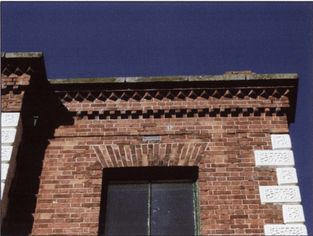
3.115: Number 11 Rostrevor Terrace: detail of parapet.
