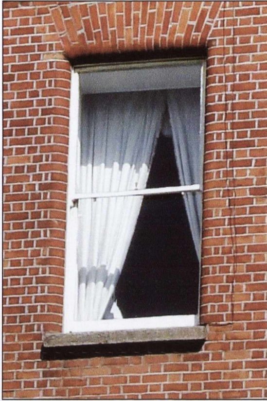
4.15: Number 4 Warwick Terrace: detail of upper floor window.
