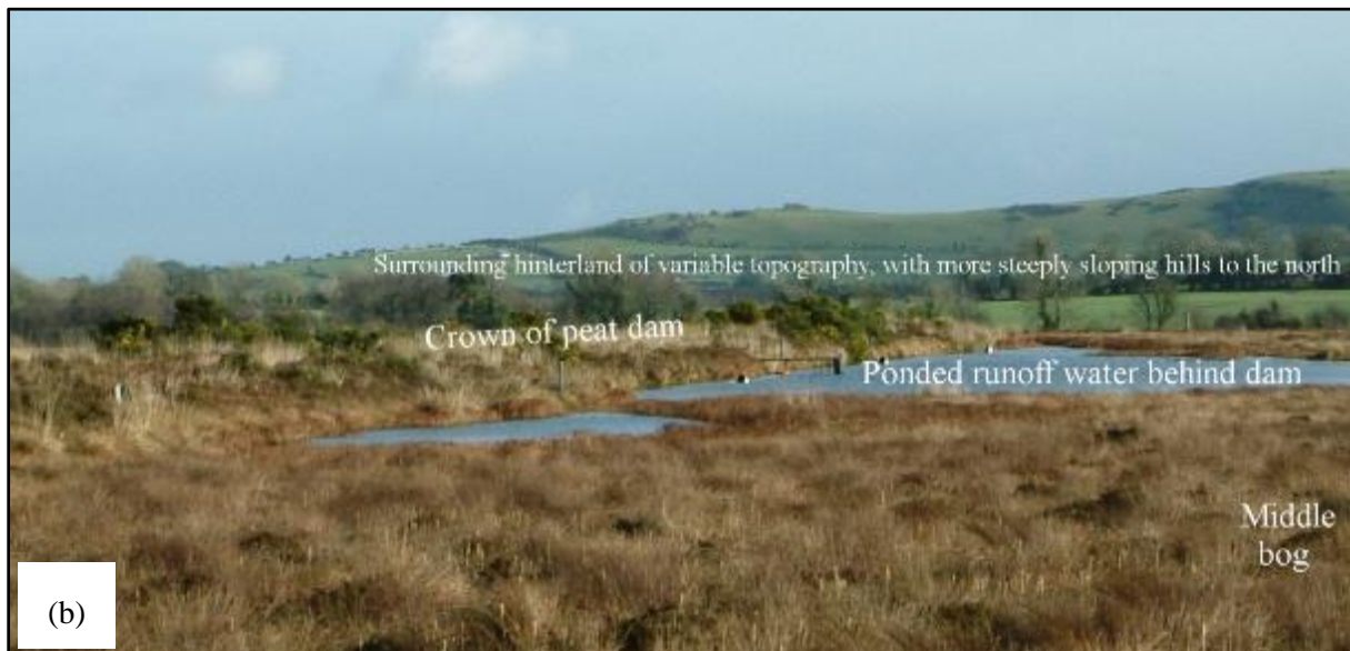
Fig. 5. Peat dam near northern margin of Raheenmore raised bog, County Offaly, Ireland: (a) schematic cross-section diagram; (b) photograph taken from high bog
