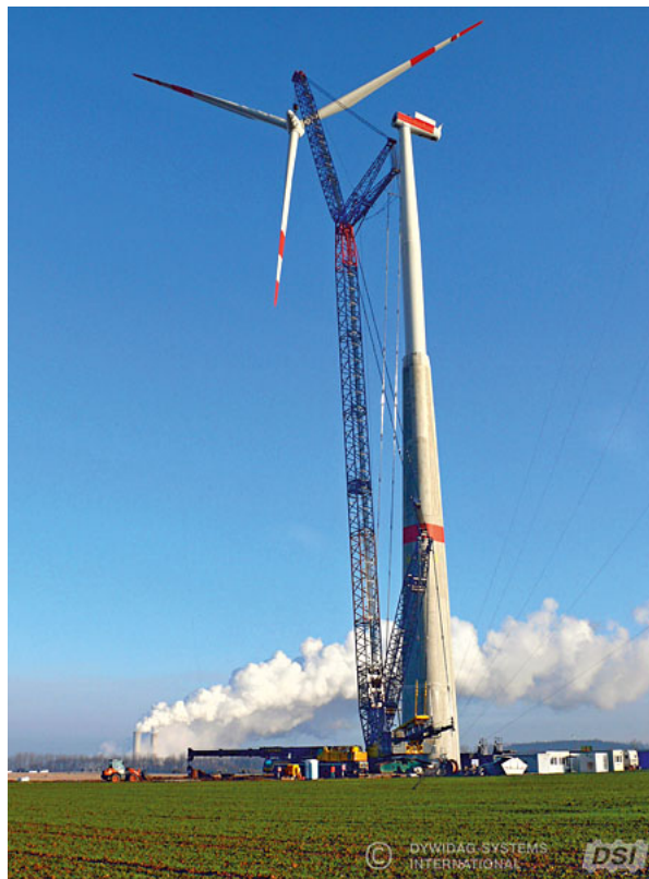
Figure 2.11: ATS Hybrid Concrete-Steel Tower
