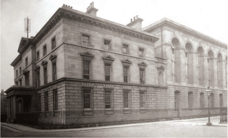
20 Exterior of the Public Record Office of Ireland (c.1914). The record house appears in the foreground (left), with the record treasury behind; between the two structures is the 'isolation space' that saved the record house from fire in 1922. The strong room, which was adjacent to the search room, is the fourth window from the left on the ground floor of the record house, identifiable from the iron bars covering the window. Photograph © NAI, 'Mills Album', presented to James Mills by his colleagues in the PROI on his retirement as deputy keeper in Aug. 1914; returned to the PROI in Feb. 1951 by his sister, Miss Mills.
