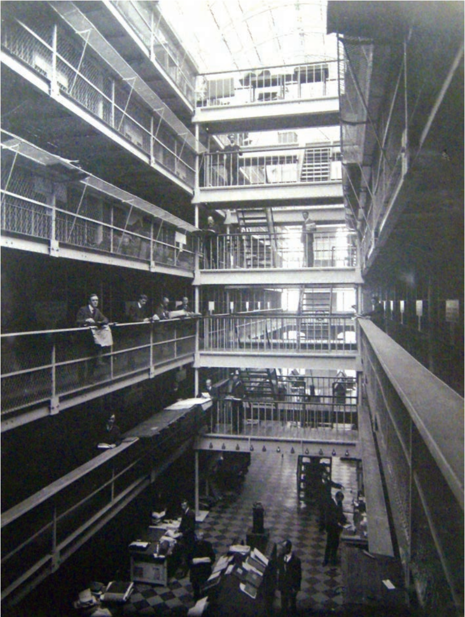
22 Interior of the record treasury, Public Record Office of Ireland (c.1914). The upper portions of the building were utterly destroyed in 1922. Now rebuilt, it houses the land registry. Photograph © NAI, 'Mills Album'.
