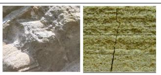
Fig. 1 Differential erosion, Drumbane sandstone
