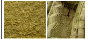
Fig. 2 Flaking, Drumbane sandstone
