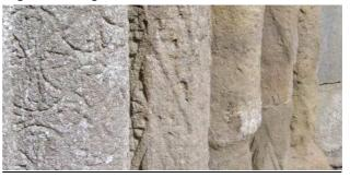
Fig. 3 Granular disintegration, Killaloe sandstone
