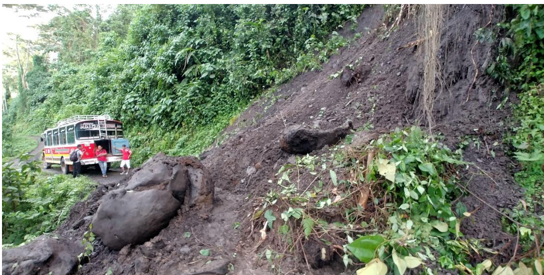
Figure 25: Photo of landslide blocking road in El Carmen de Chucurí
