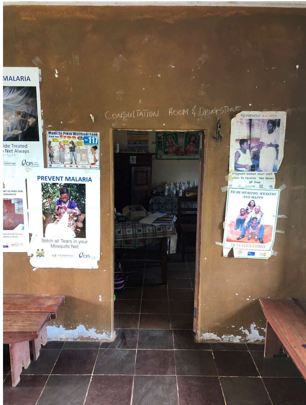
Photograph 1.3: A consultation room and drug store in Junctionla MCHP (photograph taken during fieldwork 24 July 2018)
