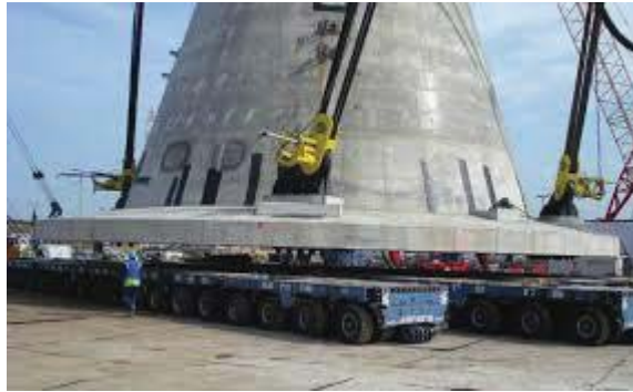
Figure 1-11: Thornton Bank, Phase I - flat based bottom GBF at quayside (Piere, 2009)
