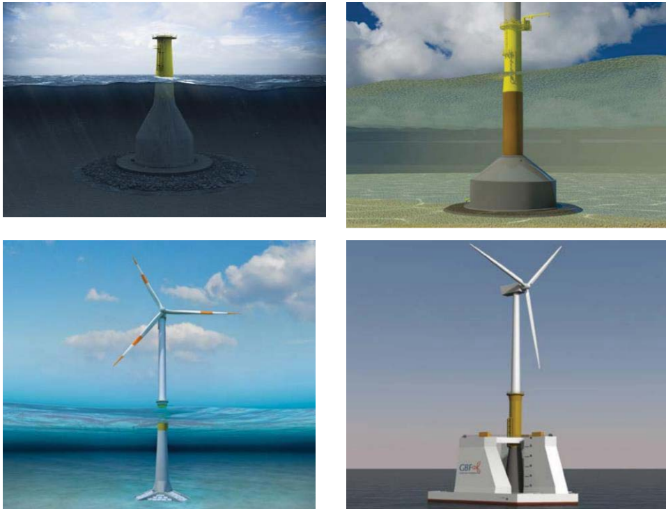
Figure 1-9: Image of other GBFs considered. Top left: Crane-Free Gravity Base (Seatower, 2013), top right: BAM Van Oord, bottom left: Strabag & Bottom Right: Ramboll, Freyssinet/BMT Nigel Gee (The Carbon Trust, 2015)
