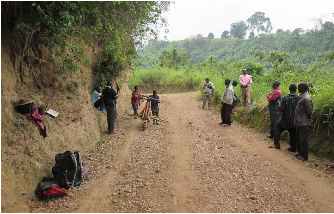
Figure IV.22: Road cutting along the side of the Ruindi river valley to the east of Kirima village at log BVγ-18.
