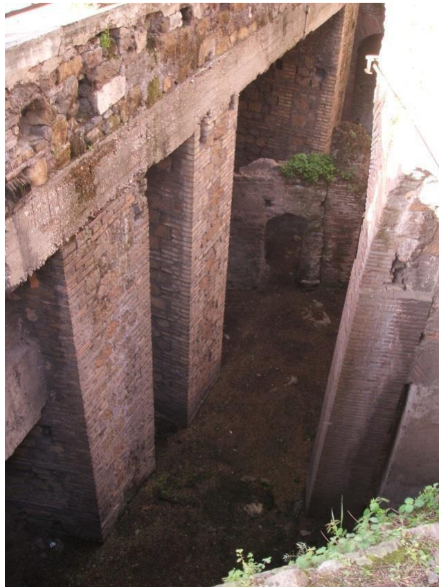
Figure 30: View of ground floor of insula Ara Coeli on slopes of Capitoline from the modern street.
