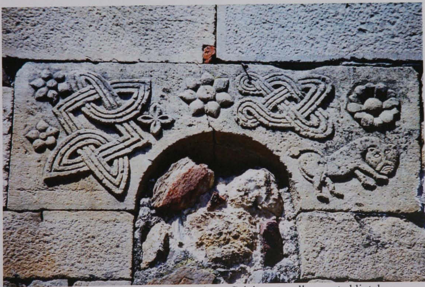
Fig. 261; Ss. Giovanni ed Ermolao a Calci, east wall, arcuated lintel.
