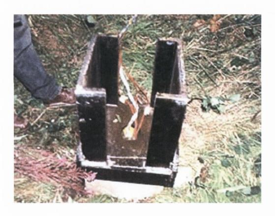
Plate 3-7: Helmet structure located over pile AL1
