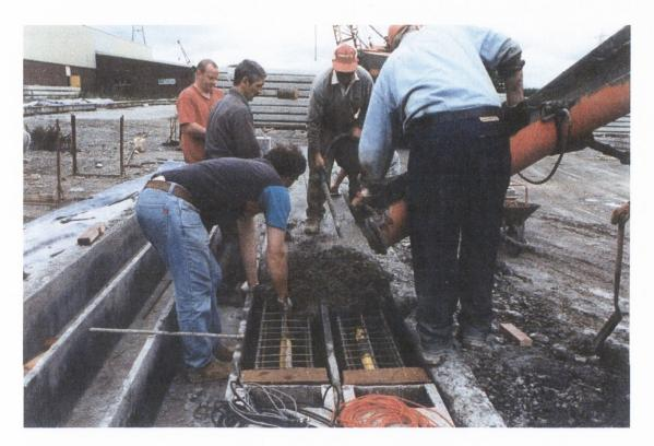
Plate 3-6: Concrete placement
