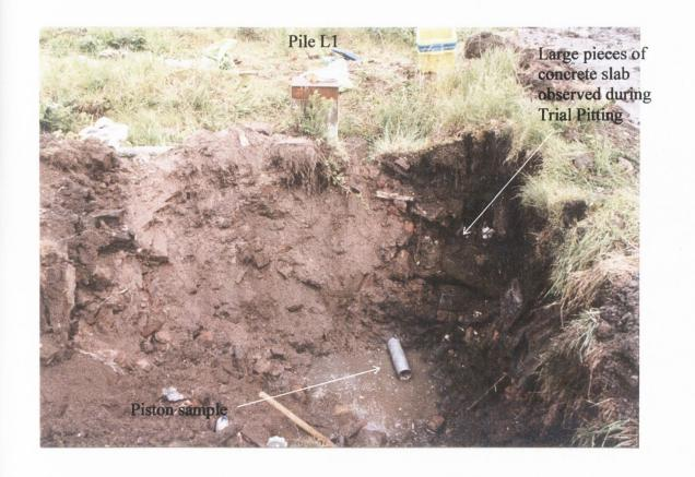
Figure 5-15: Trial pit excavated around pile L1 revealing large pieces of concrete slab
