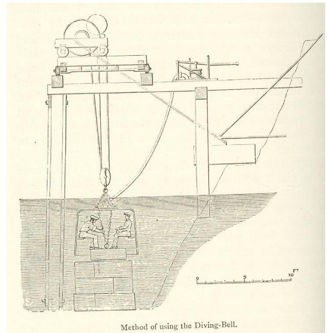
Figure 3. Section of Rennie’s diving-bell building the base of a (vertical section) pier.
