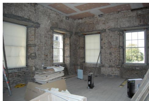
Figure 2. Interior of building prior to the application of insulation.
