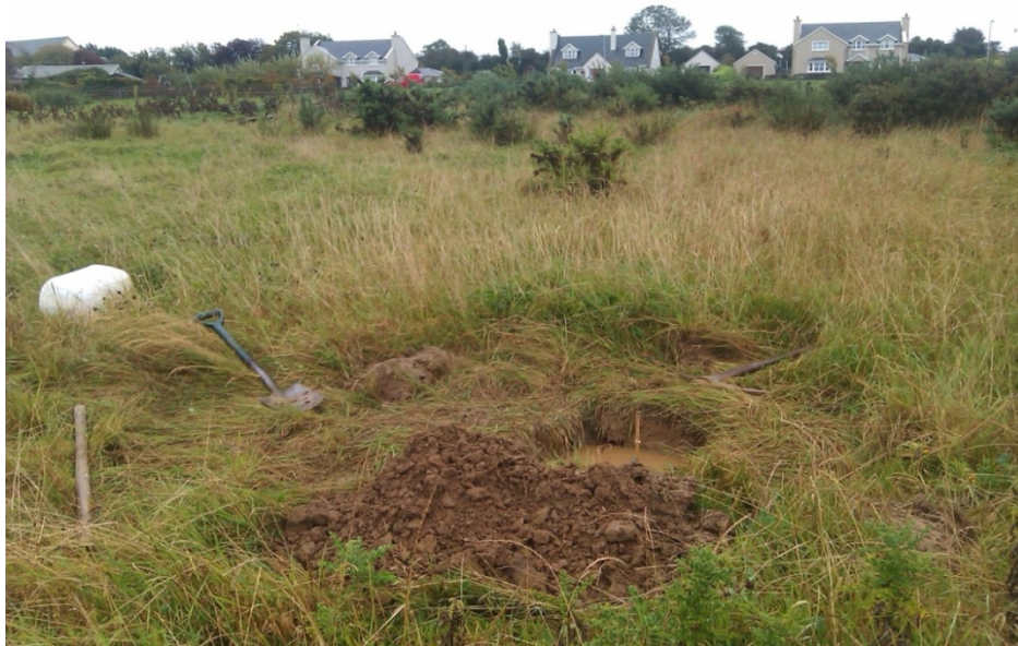
Figure 5.4 Percolation Test at Carrigeen, Co. Kilkenny
