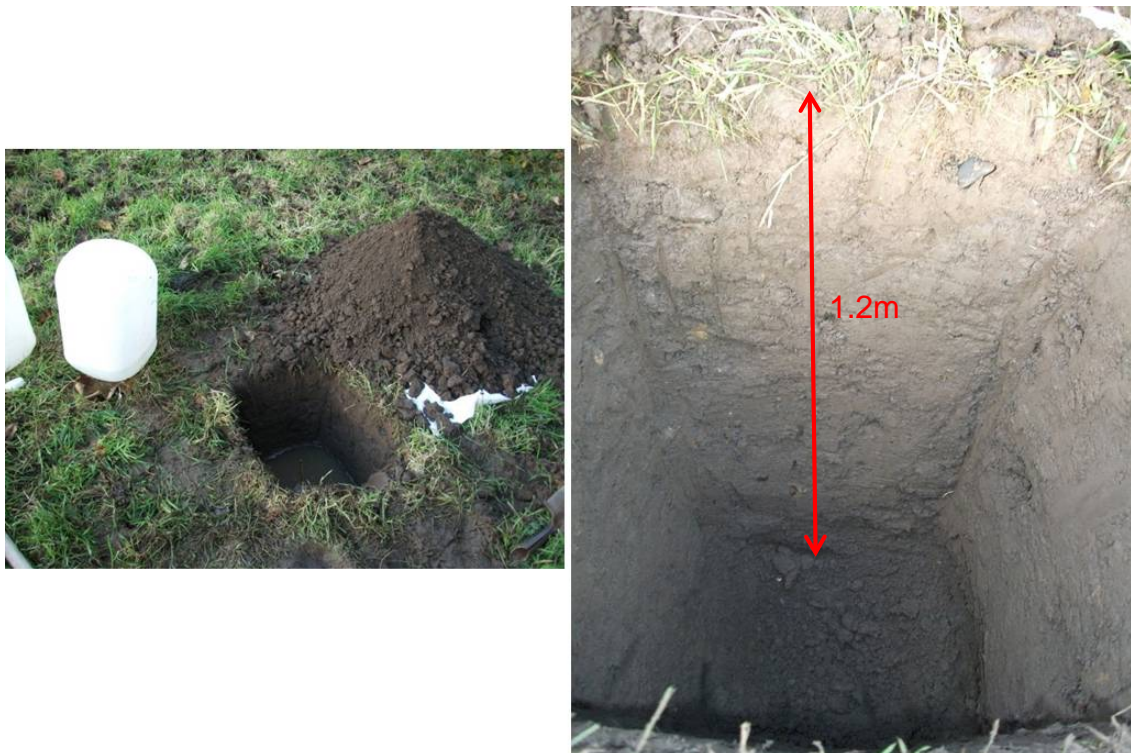
Figure 5.1 (a) Percolation Test and (b) Soil Profile at the Naul, Co. Dublin
