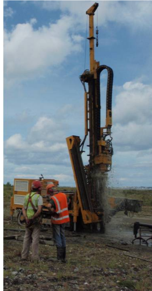
Figure 4.11 (a) Typical Nested Piezometer Setup. (b) A Borehole being drilled with Beretta Rig
