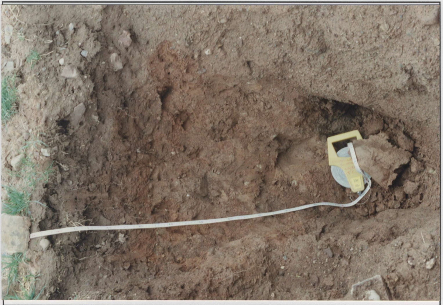
Plate 4.2 Trial pit dug in plot 5, which contains borehole 2.
