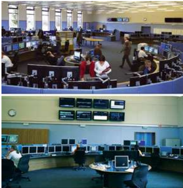
Figure 9.2: Consoles in the CERN Control Centre for monitoring and control of the LHC apparatus.
