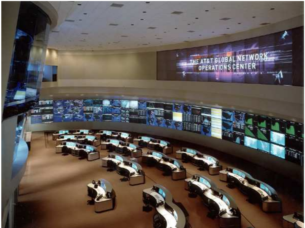
Figure 9.1: The videowall at the AT&T global network operations centre, one of the largest command and control centres in the world. One hundred and forty-one rear-projection video screens are employed, each measuring 1.2 by 1.5 meters.
