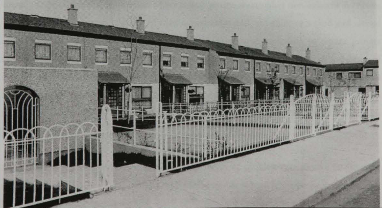
Plates 8.10 – 8.12 Darndale Refurbished
