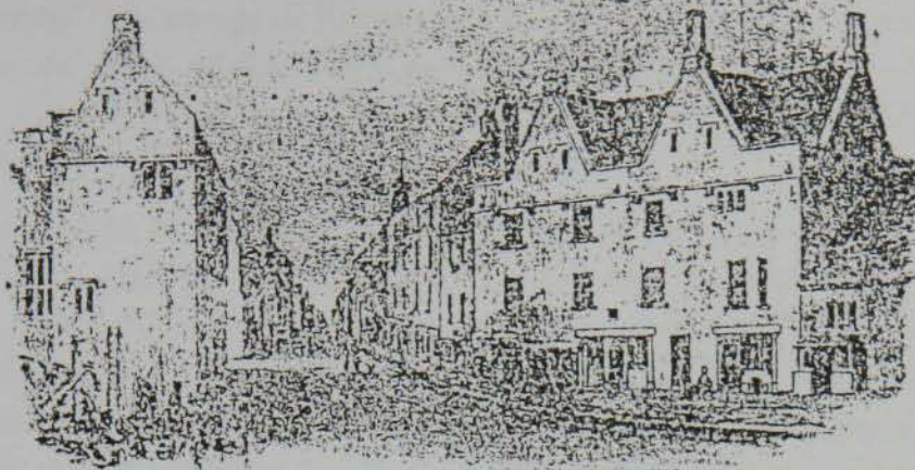
Old Houses of early modern date still standing in the High Street, Kilkenny, in the mid-19th century
