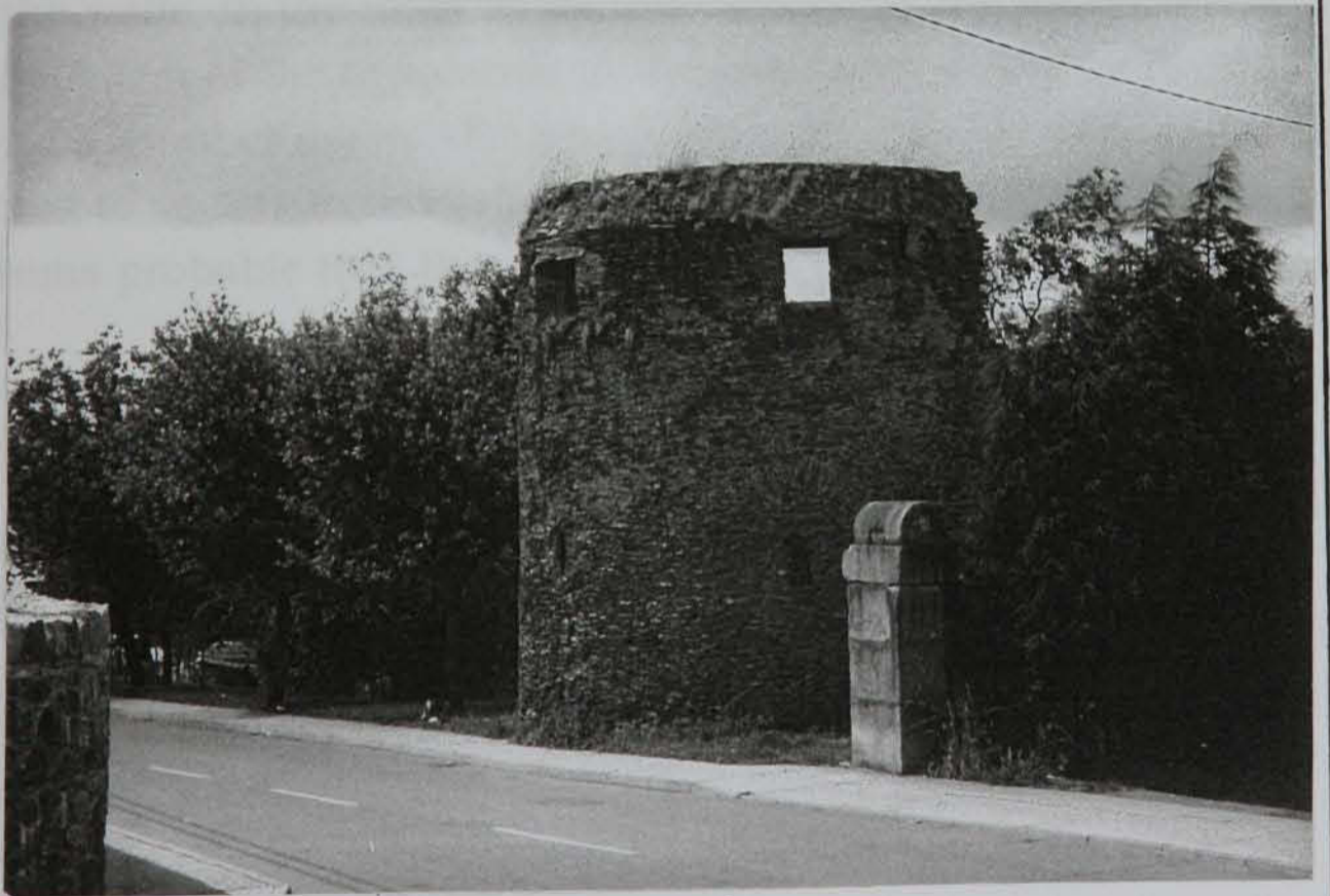
Fig. 75. The only surviving mural tower at New Ross.
