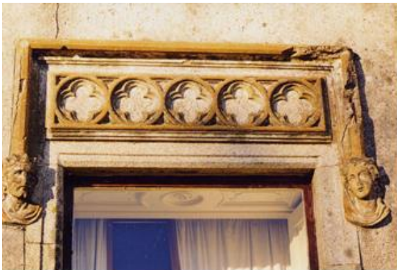
Figure 1. Borris House, County Carlow, a 19 th century building with Roman cement mouldings.
