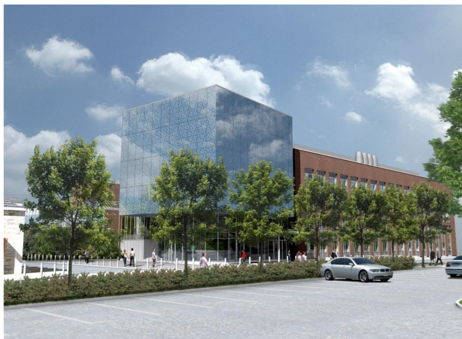
Figure 2 SSPC headquarters at the 15,100m 2 Bernal/MSSI Complex, University of Limerick
