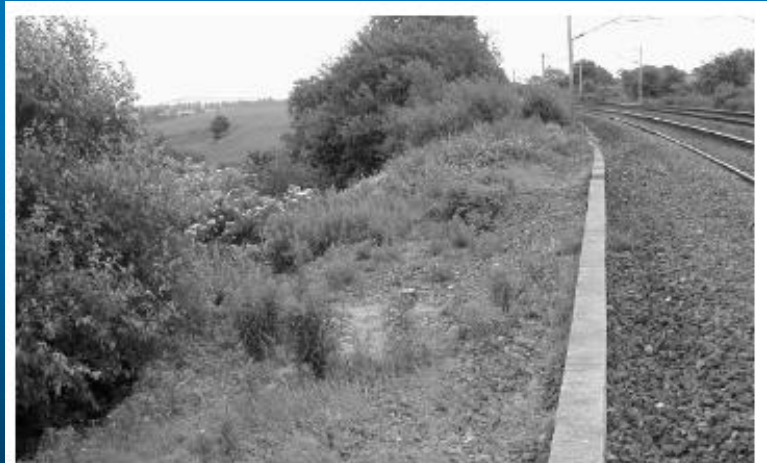
Figure 3. View southwards along Up-line slope.
