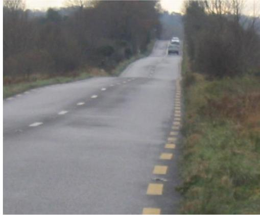
*Figure 2: Extreme undulations on the rampart road of the N62 national secondary road, County Offaly, Ireland.*
