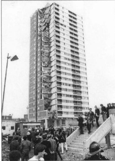
*Fig. 1: Ronan Point apartment tower after collapse*
