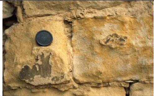
Figure 9- Masonry damage enhanced by mixing permeable sandstone with impermeable OPC mortar. Abalos Church, La Rioja, Spain.
