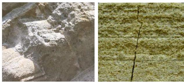
Fig. 1 Differential erosion, Drumbane sandstone
