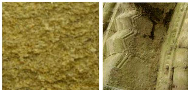
Fig. 2 Flaking, Drumbane sandstone
