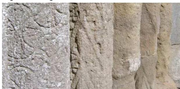
Fig. 3 Granular disintegration, Killaloe sandstone
