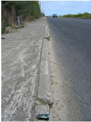
Figure 6. Deployment on a two-way single carriageway
