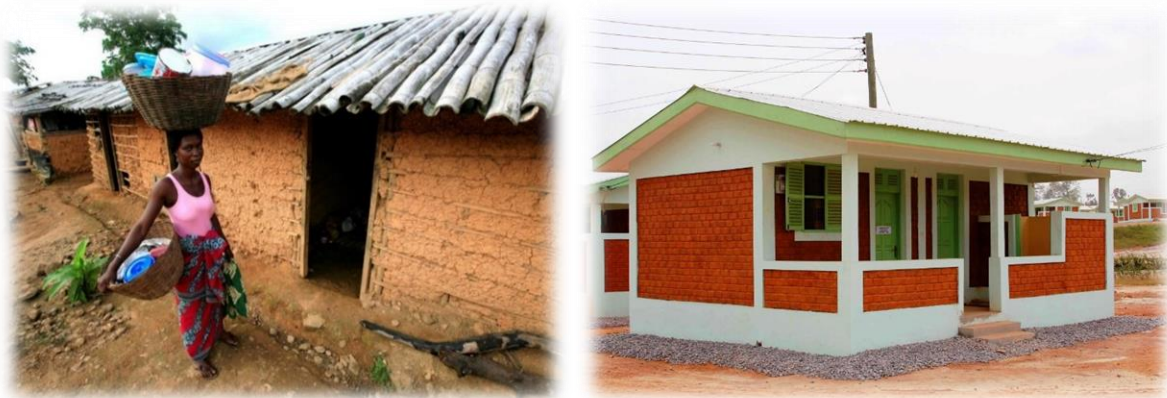
Figure 4.9: Images of the nature of buildings in Old and New Salman. Source: Adopted from Cision (2012).
