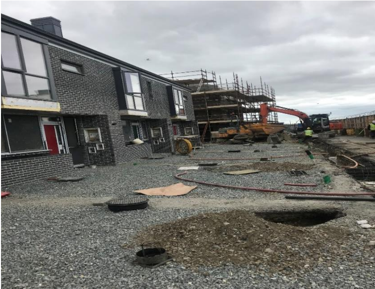
Figure 3.6 Houses at Location 1
