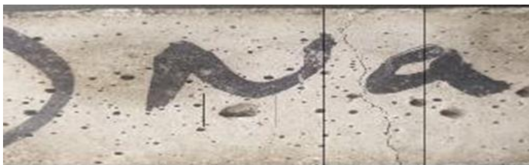
Figure 5-6 NaOH activated GGBS, 60°C-cured, after salt crystallization cycling showing cracks.
