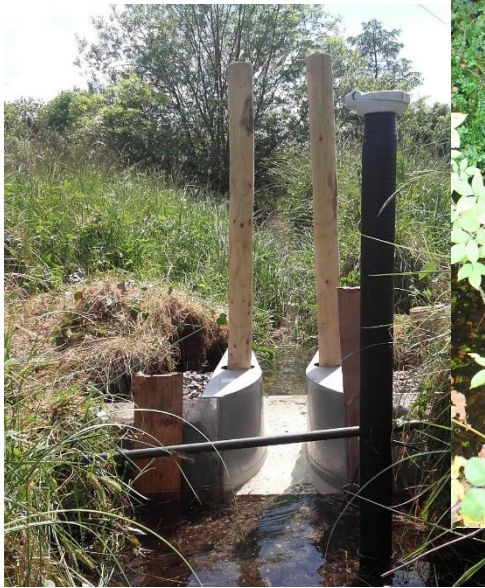
Figure 4.8. Ballymore hydrometric station and flume.
