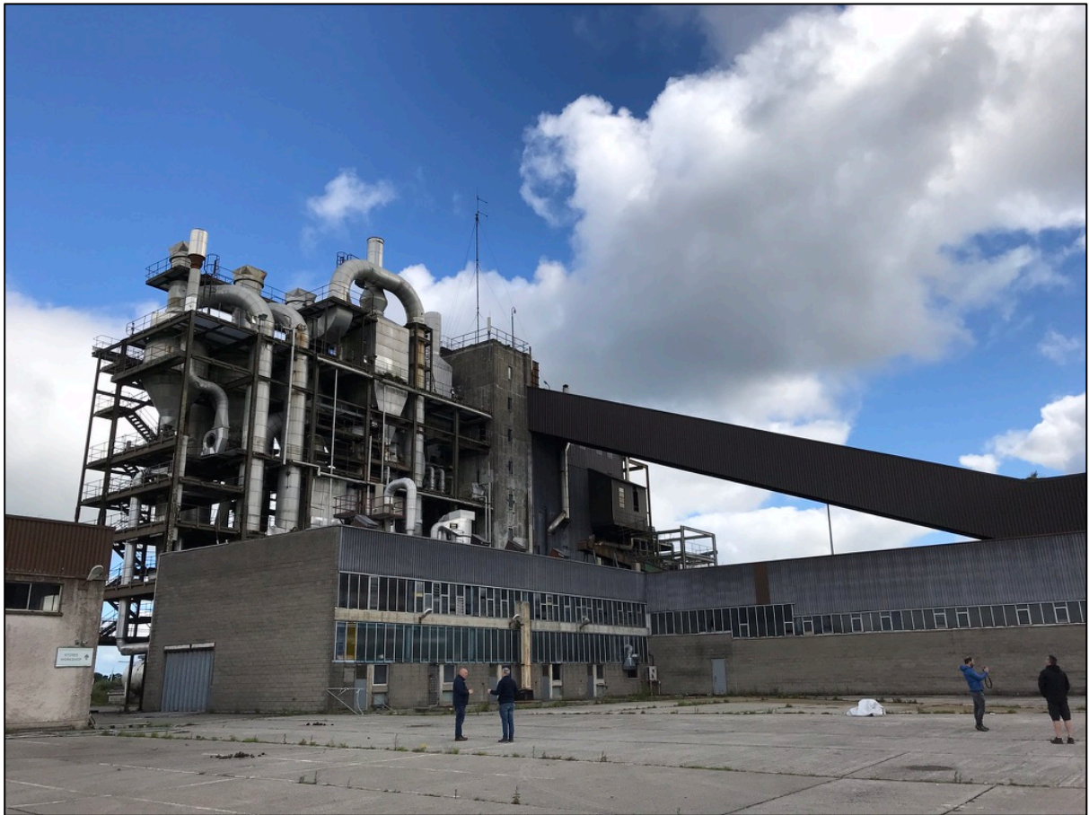
Plate 12.6 Littleton briquette factory in July 2020, undergoing transformation into as a plastics recycling facility.
