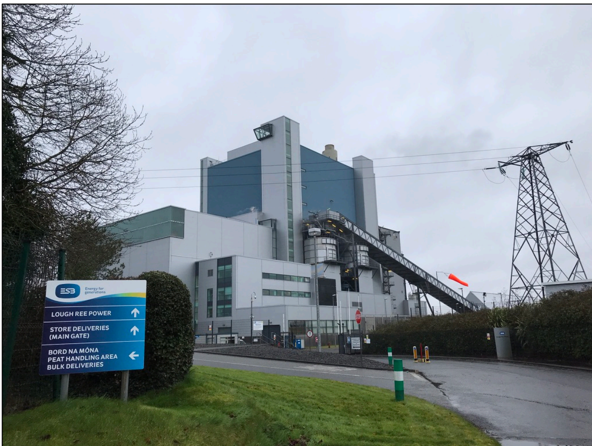
Plate 5.4 ESB Lough Ree power station, Lanesborough, Co. Longford This image was taken in March 2020, in the months prior to its closure.
