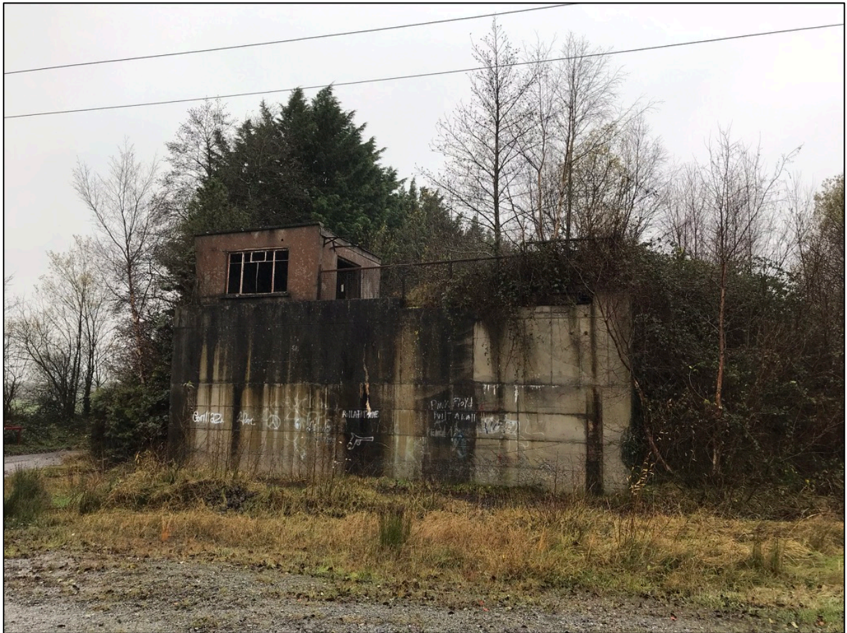
Plate 5.2 A tip-head, Co. Offaly This derelict facility once enabled the loading of vehicles with peat from above. Relics of the peat industry past can be found across the Irish midlands and are instructive of its slow decline.
