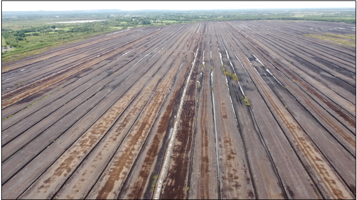
Plate 4.7 A post-industrial Bord na Móna bog, Co. Longford This bog is part of the BnM Mountdillon group. The striation in the landscape are drains that were dug to remove water. With no vegetative cover present or food available, these spaces are unsuitable for animal life. Following rehabilitation, flora and fauna re-emerge.
