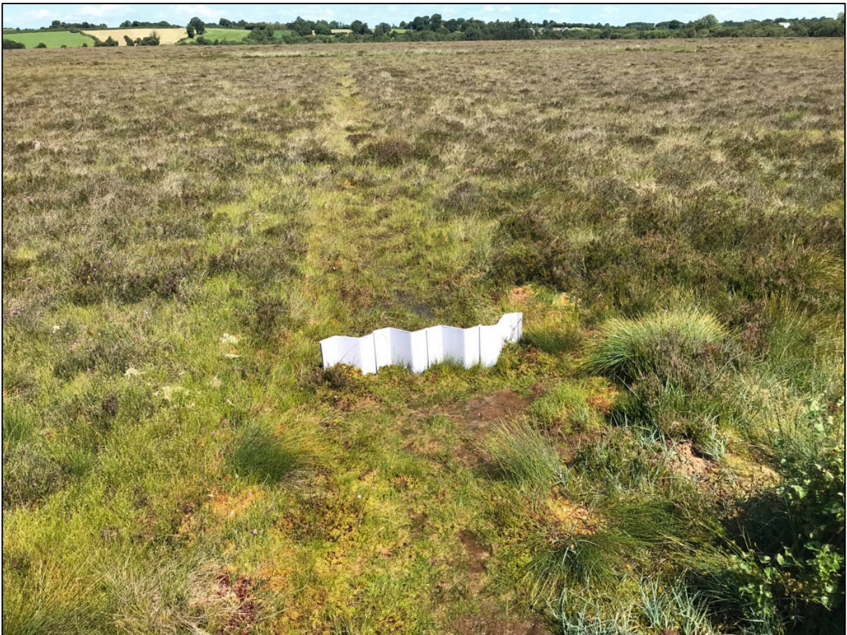
Plate 9.3 Drain-blocking dam This plastic apparatus blocks an old drain previously dug into Clara Bog SAC.
