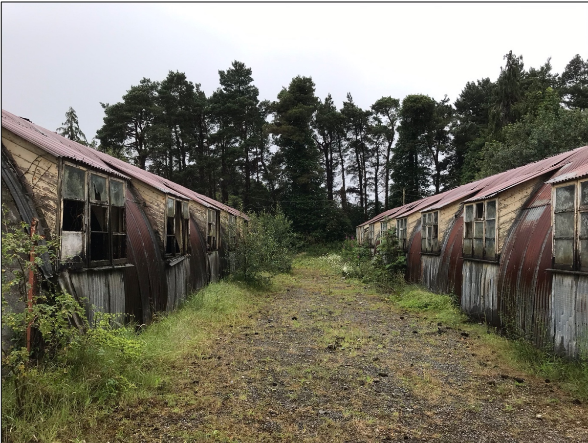
Plate 12.4 Derelict housing Rows of BnM Nissen huts adjacent to the company’s Boora offices. These structures used to house workers during the early days of the peat industry. Today, they lie abandoned.
