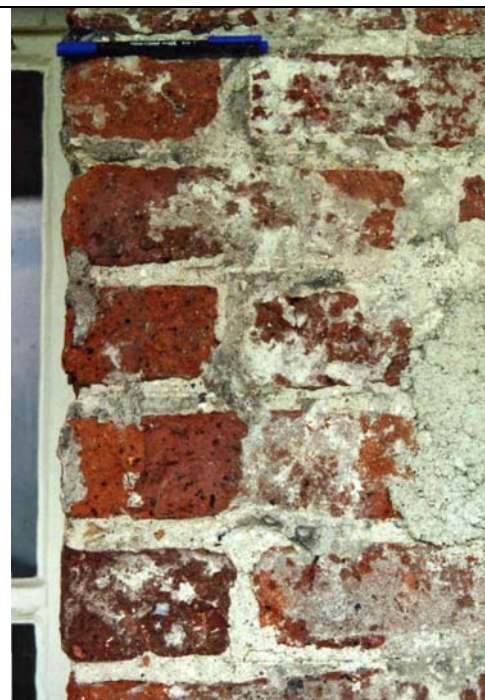
Figure 3- Detail of brickwork and lime mortar (East elevation).
